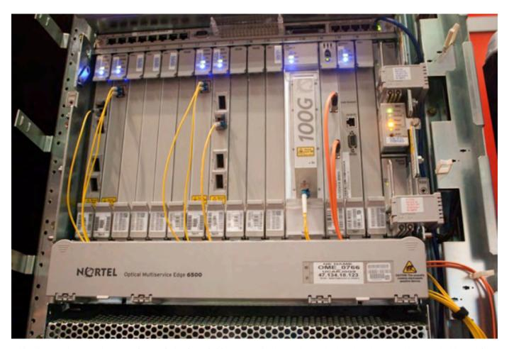
This picture shows a close up of one of the OME6500 systems in the racks at the booth. The only thing needed is two free slots in an OME6500 to put in a 100Gbit/s transponder. The 100G links operate on the existing 10 Gbit/s optical wavelengths. In July 2009 Nortel and SURFnet successfully demonstrated that this works in its live network over a distance of 1244 kilometers on its link between Amsterdam and Hamburg.
